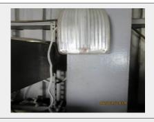
N.C: There is one light sources (1 out of 12) of emergency in the 2F production area was malfunctioned.
