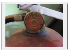
NC: There is one (1 out of 23) fire extinguisher with lower pressure in production area.
